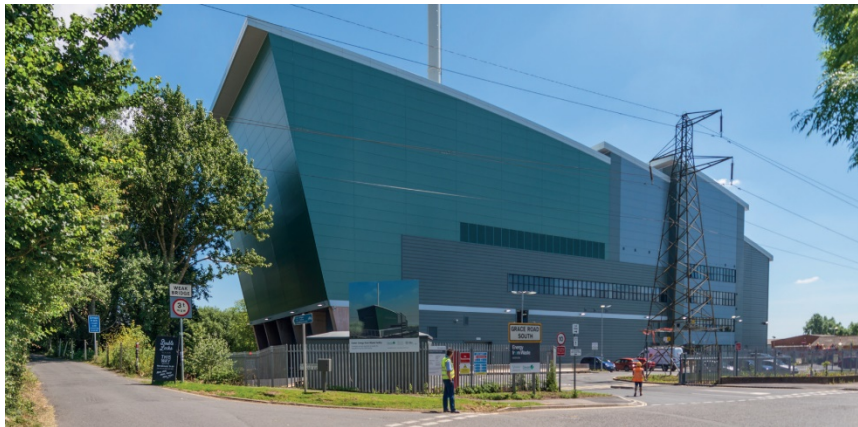
Figure 23: Exeter Energy Recovery Facility
